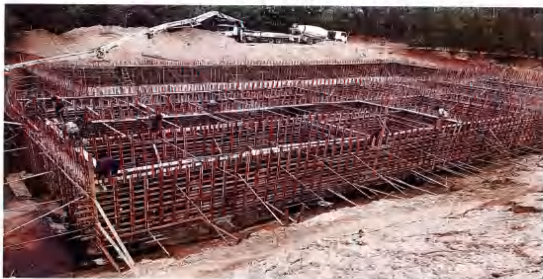
污水池立墙注入商混
